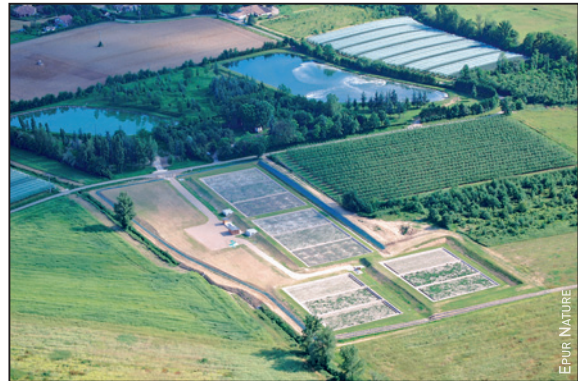
Figure 2. Station de Nègrepelisse (Tarn-et-Garonne)
